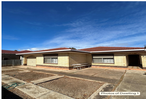
Photos of Dwelling 1
