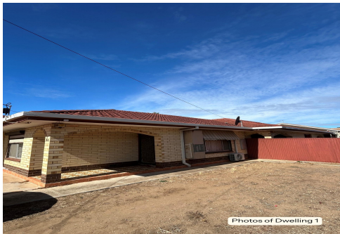
Photos of Dwelling 1
